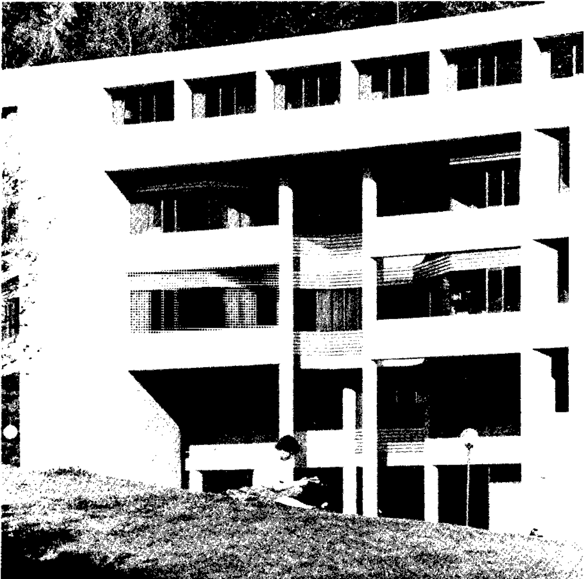
Arntzen Hall on south campus.
